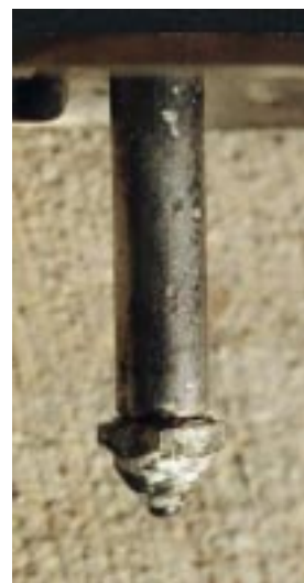
Polygon Feed as on post-1920 lamps.
