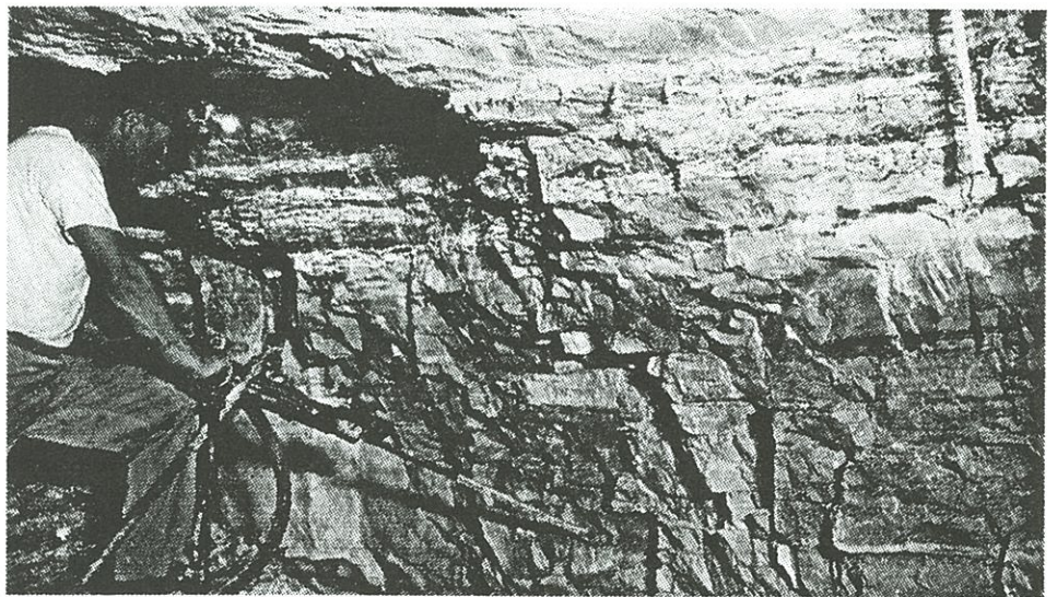
Drilling the stopes.
